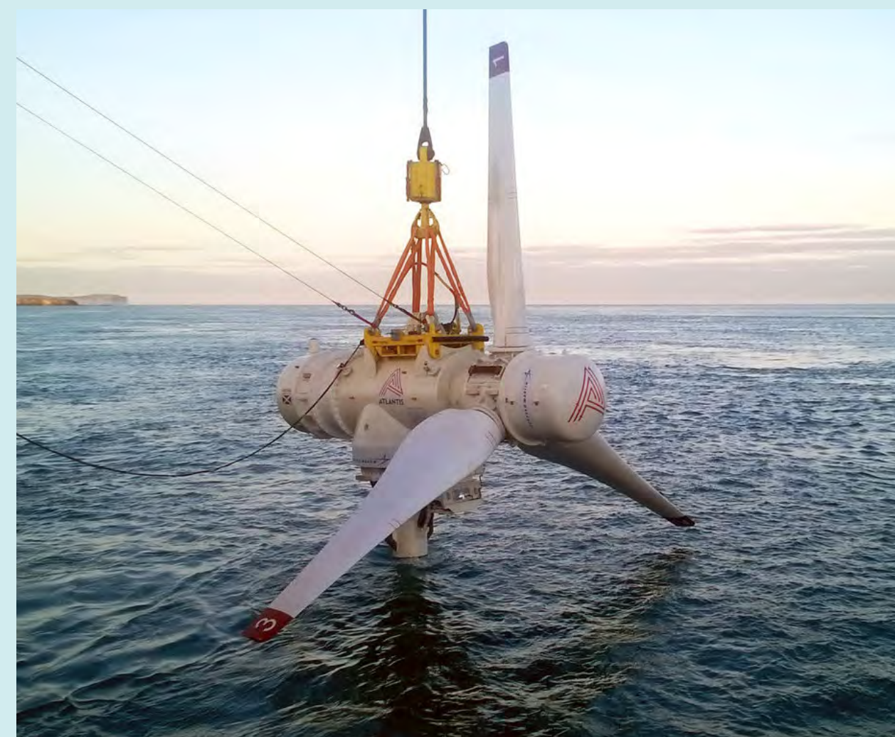
AR1500 turbine being deployed by MeyGen (Credit: SIMEC Atlantis Energy)
