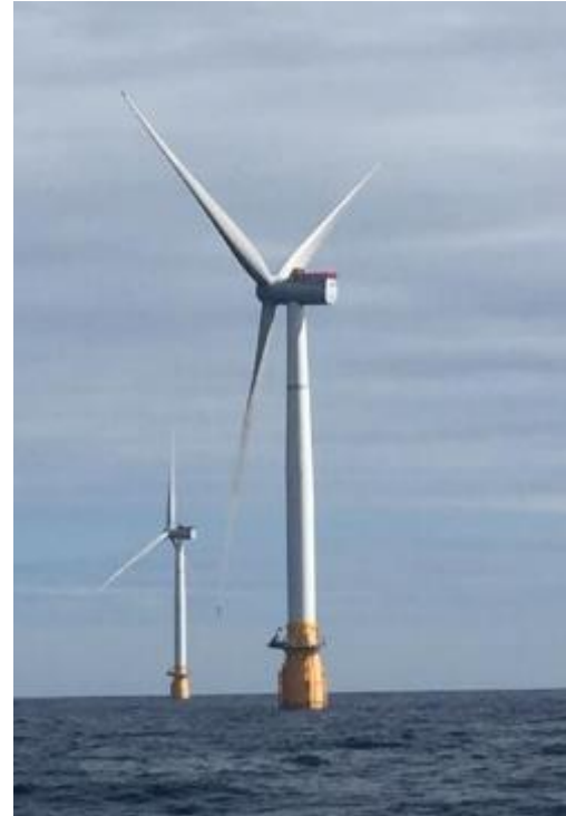
Equinor – 6.0 MW Turbines in Peterhead Scotland Hywind-2 Spar Substructures (photo credit: Walt Musial)
