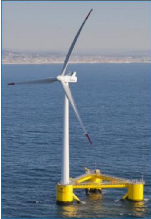
Principle Power – 2.0 MW Turbine in Portugal - 2011 WindFloat Semisubmersible Substructure (photo credit: PPI)
